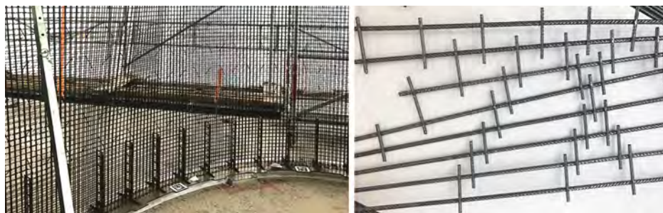
FIGURE 4.11: Insertion Experiments. Left: the regular-spaced straight bars in the Mesh Mould project; Right: the fabricated experiments to obtain data for the computational system.
