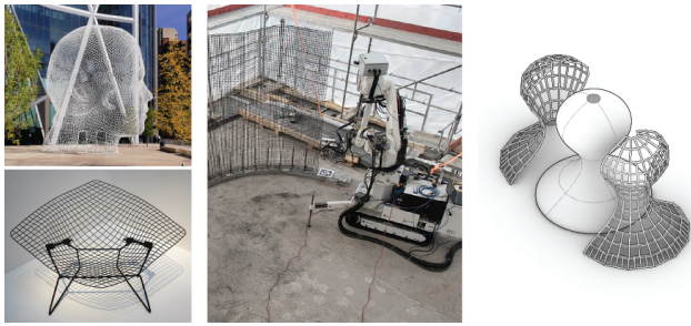
Figure 2: The 12-meter tall metal frame sculpture “Wonderland” by Spanish sculptor Jaime Plensa and the Diamond Chair design by Harry Bertoia (left). Robotically-constructed rebar for concrete applications (Mesh Mould [HLGK15], middle). Regular structures are insufficient to achieve high curvature detail, and it is unclear how to decompose complex shapes into fabricable units with globally aligned bar structures (right). Lower left image by Sandstein; license: Attribution-ShareAlike 3.0 Unported.
